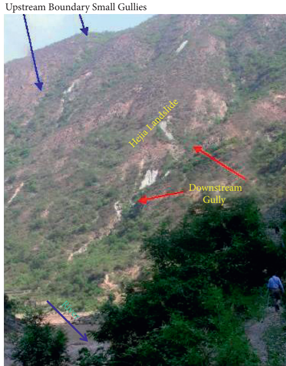
FIGURE 8: Downstream gully and downstream boundary of the Hejia landslide.
