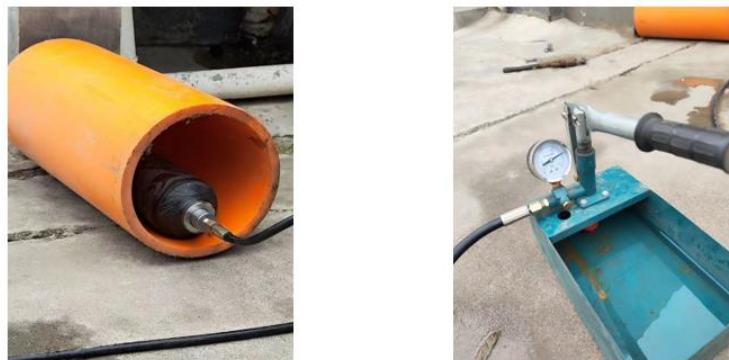
Fig. 7. Pressure test of ballast tank
