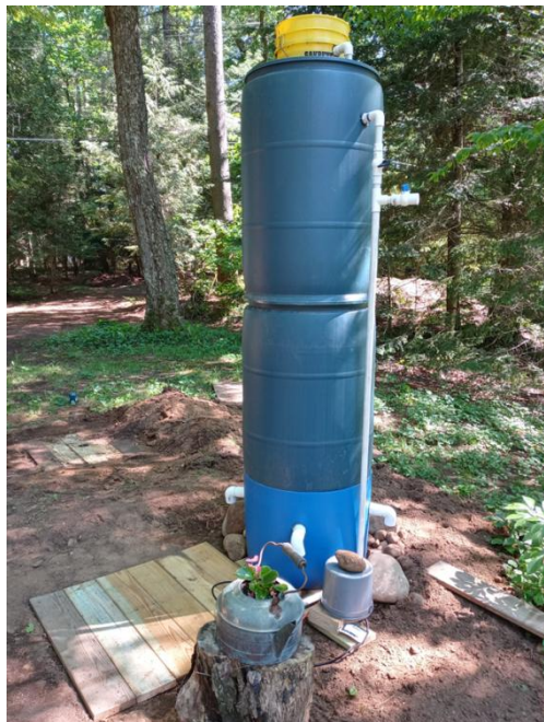
Fig. 5. Field Bio-tower Septic (FBTS) System Installation [28]
